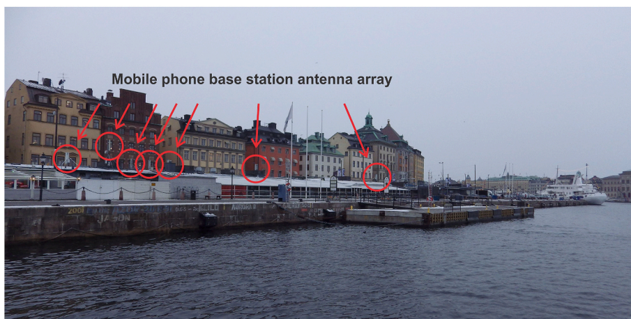
Fig. 5. The antennas are mostly facing the buildings, as the operators want to force the wave into the old town through the narrow streets. Considering the low placement of antennas and pushing all this power - creates very high exposure levels nearby.
